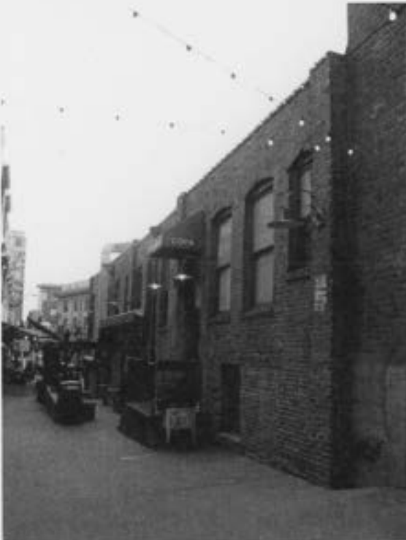
Dec 2009 View south Post Alley/east elevation [CKK]
