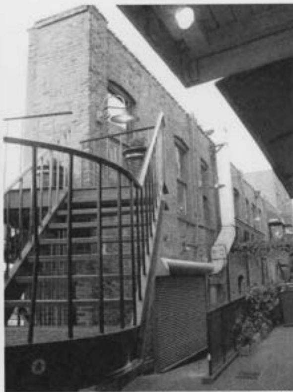
Dec 2009 View north Post Alley/east elevation [CKK]
