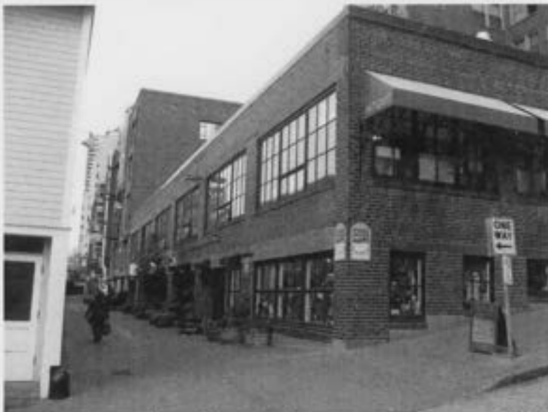
Dec 2009 - Post Alley at West elevation
