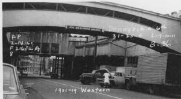
1961 - Original Desimone Bridge in foreground [PSRA]
