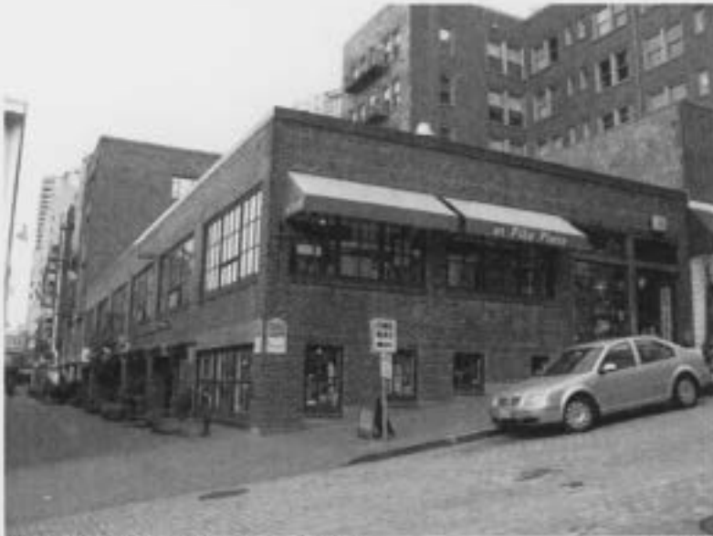
Dec 2009 - West & South elevations
