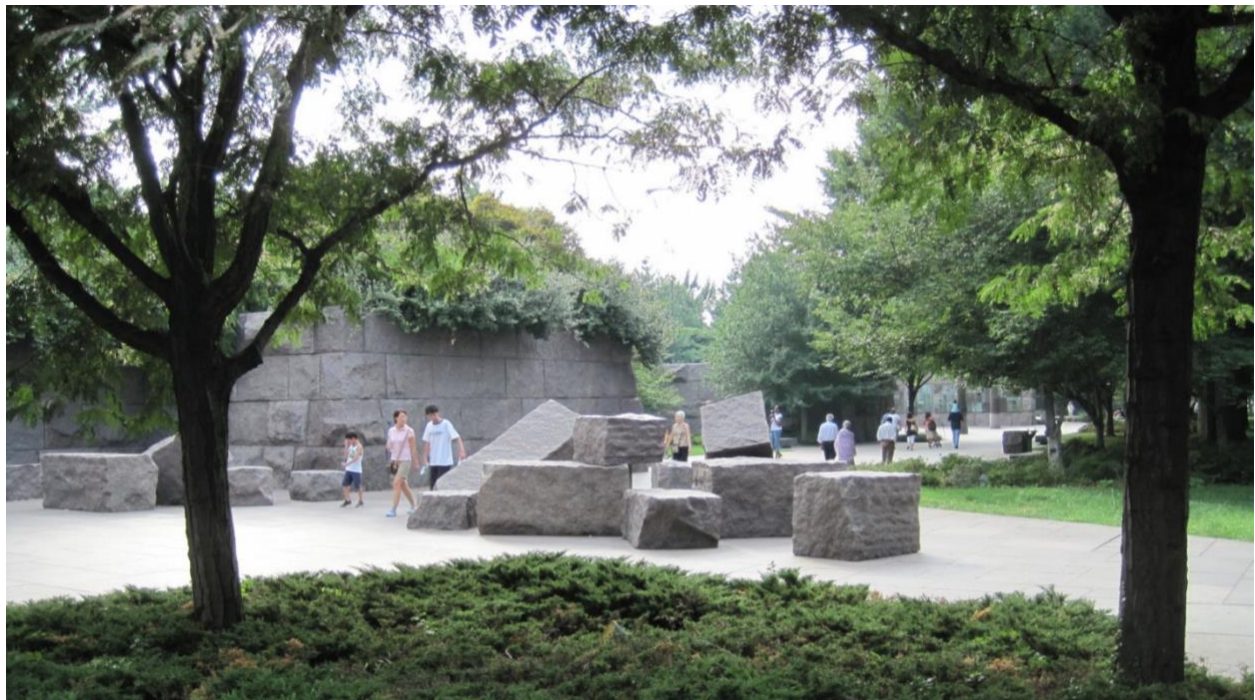
Figure 5: Built elements at Halprin’s F.D.R. Memorial, Washington, D.C., break from the strict use of right angles at purposeful moments to secure the visitor’s attention. (Charles A. Birnbaum, photo 2020)
