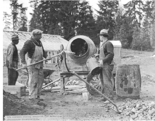
Figure 4. WPA Construction photograph, 4/16/37, showing construction of the greenhouse. Source: MSCUA.
