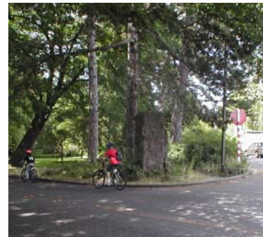
Entry Sign missing from Madison pylon, summer 2003
