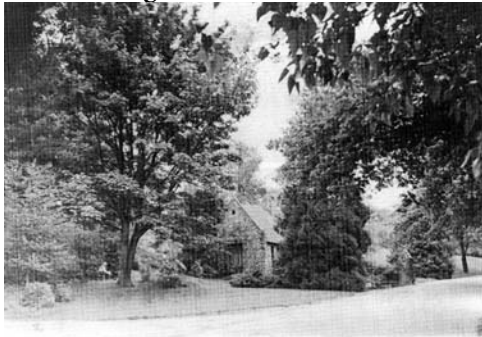
Ca. 1938 north façade (MSCUA 379/1/11)
