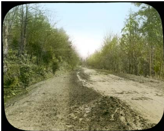
Figure 7. Azalea Way Before Improvement. Asahel Curtis glass slide of Olmsted Brothers Photo, 1934. Source: Arboretum.
