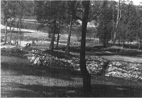
WPA Installing Drainage in Glen, 1938 (MSCUA 379/1/2)
