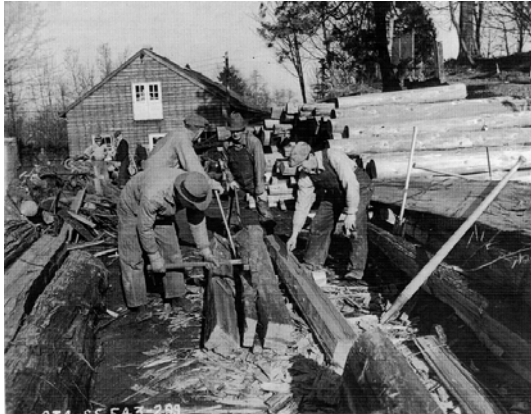
Figure 3. WPA Construction photo, 1/28/36, showing the east fence, and the barn. Source: MSCUA.
