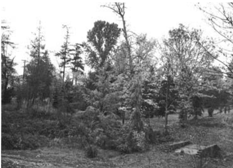
Looking West Across Boulevard at Stone Bridge, ca. 1950 (Arboretum)
