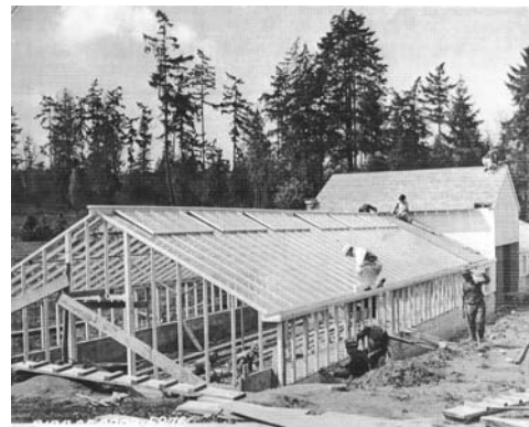
Figure 7. Construction of Potting Shed with Greenhouses, March 16, 1937. Source: Arboretum.
