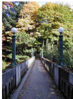
View to the east on the bridge, spring 2003
