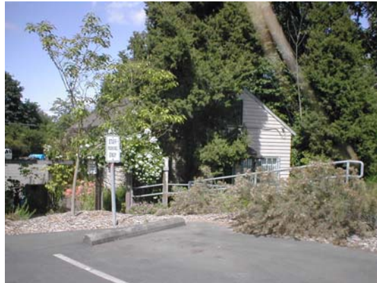
Maintenance Building obscured by Vegetation, summer 2003
