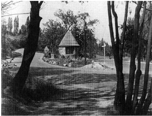
Figure 10. The stone kiosk at the intersection of Interlaken and Lake Washington Boulevards, ca. 1938. Source: MSCUA.
