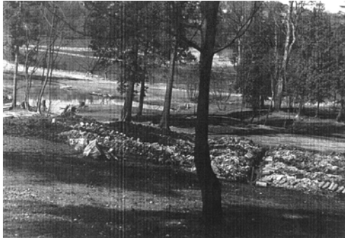
Figure 16. Installation of drainage system in Rhododendron Glen in 1938. Source: MSCUA
