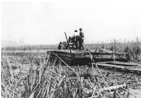
Figure 12. Dredging Lagoons, ca. 1938. Source: Arboretum.
