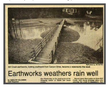
Secondly, the Department of Ecology, which is responsible for the safety dams, has concluded that the Mill Creek Earthworks Dam is not adequate for the safety of the city of Kent during a 10,000year storm event. Though this seems like an outrageous number to design to, the DOE has maintained such standards for all its dams based upon the number of people who could possibly die if the dam were to collapse under such
